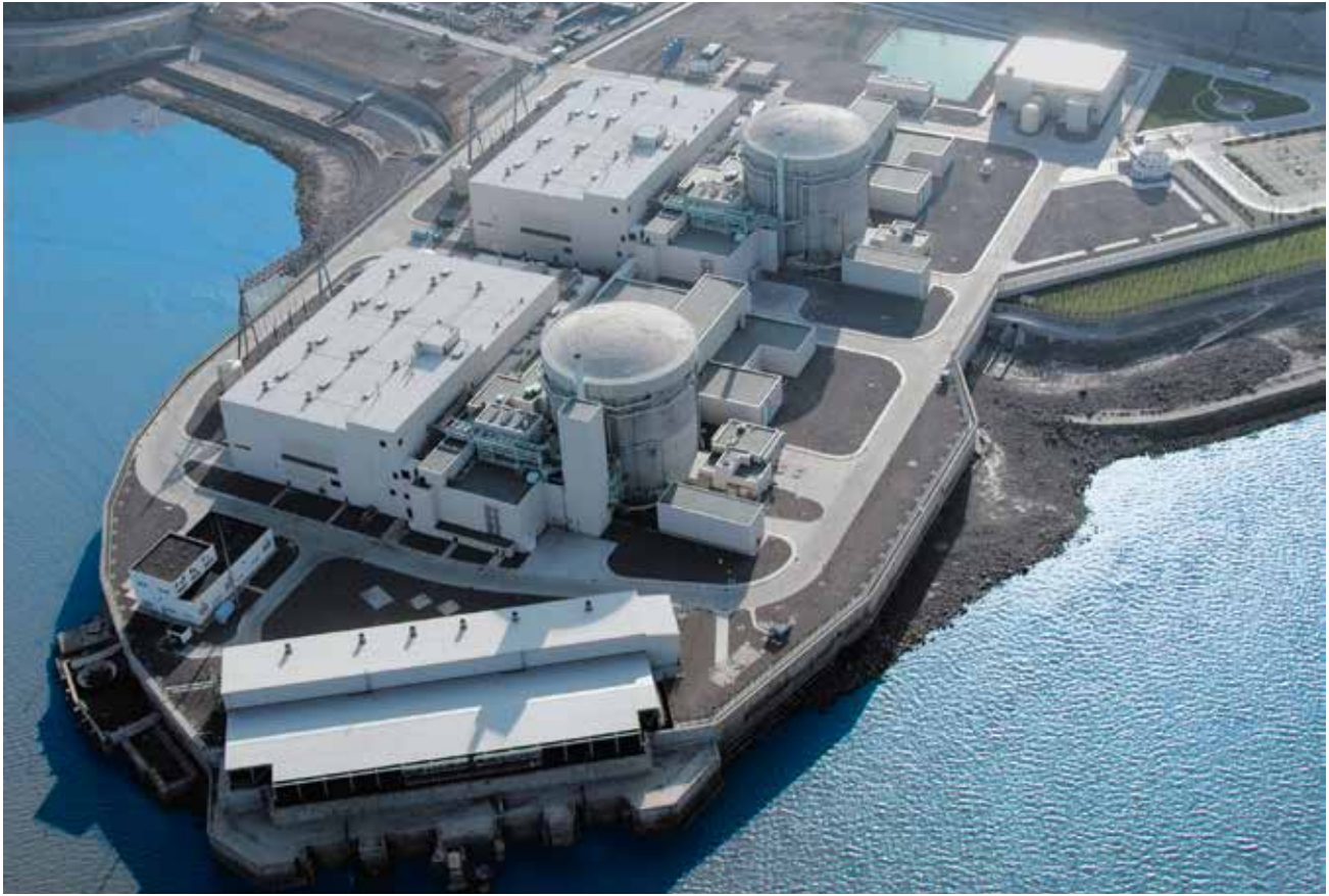
Qinshan CANDU Reactors in Haiyan, China
