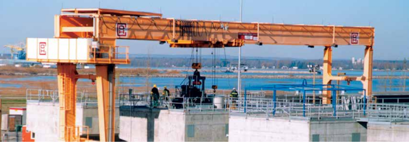
Modular Air-Cooled Storage (MACSTOR®)
