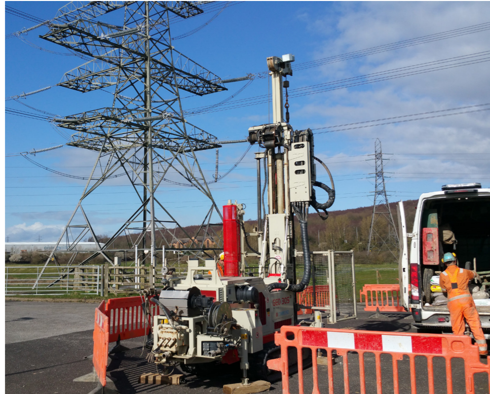
Figure 10 - Example ground investigation
